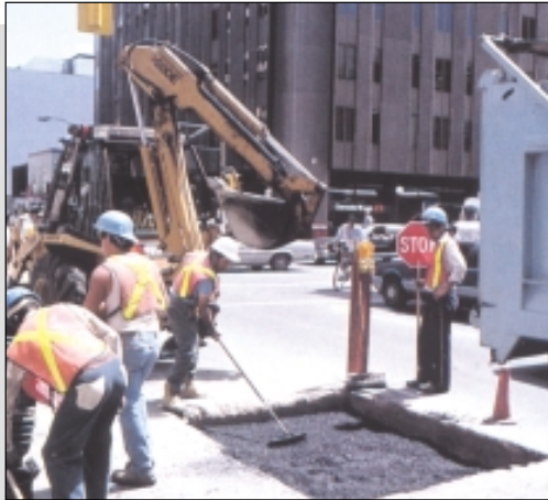
Workers move quickly to minimize any inconvenience during construction.
