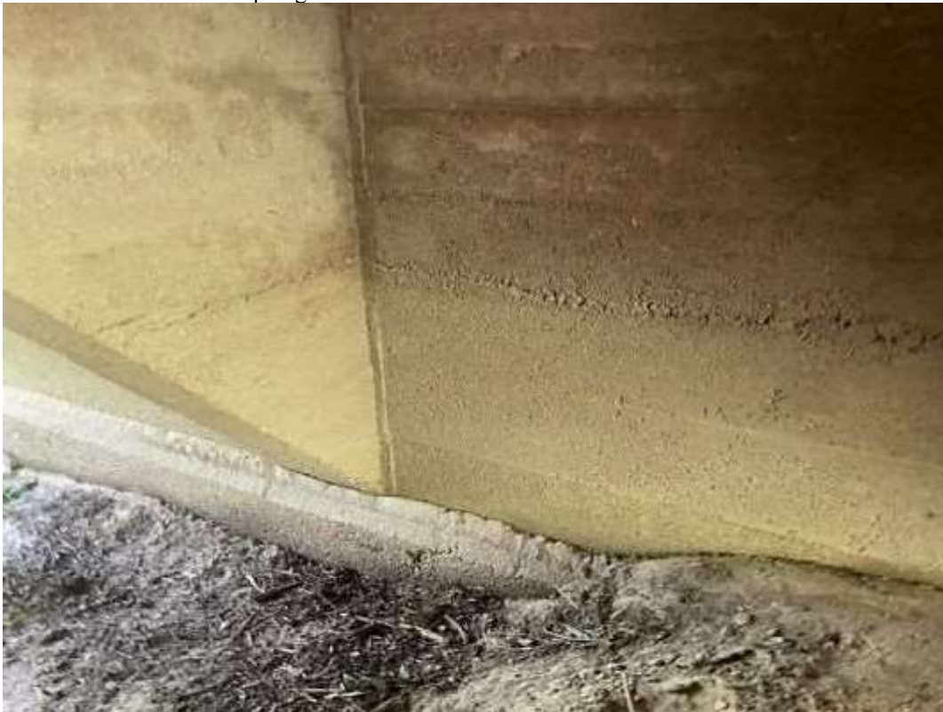
Photo 1: North foundation at end diaphragm.
