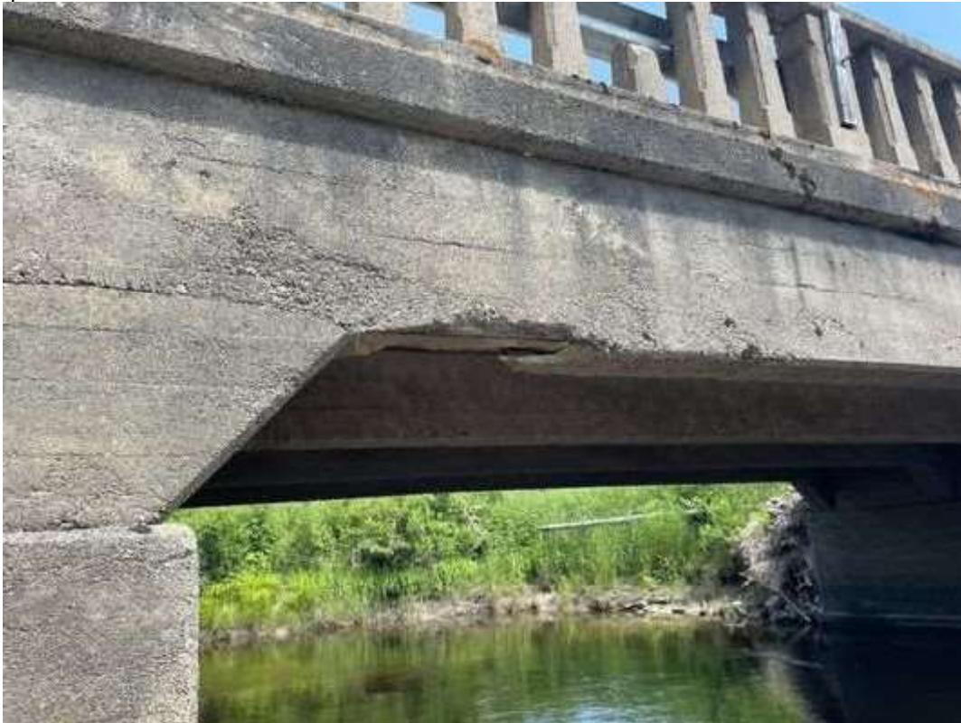
Photo 3: Spall at west side.
