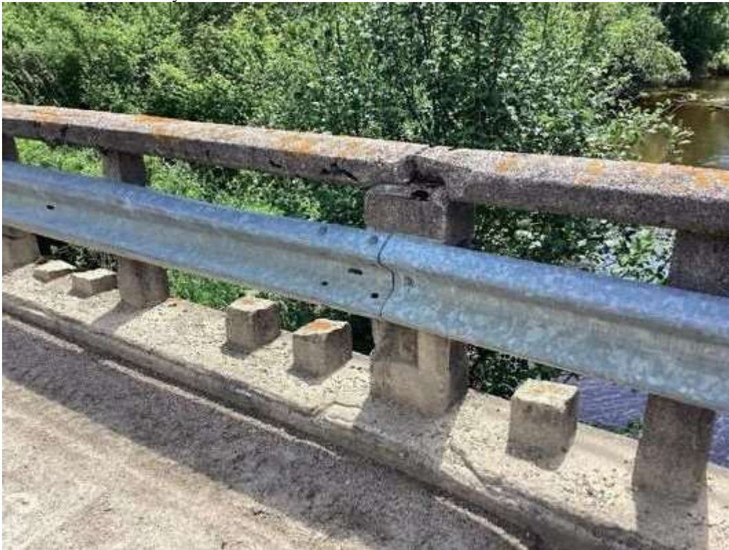
Photo 1: West Concrete Barrier System.
