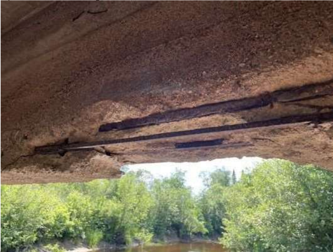
Photo 5: Exposed rebar at south girder haunches.
