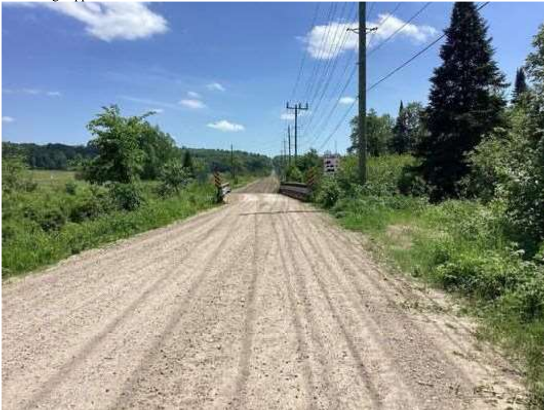
Photo 1: North bridge approach.
