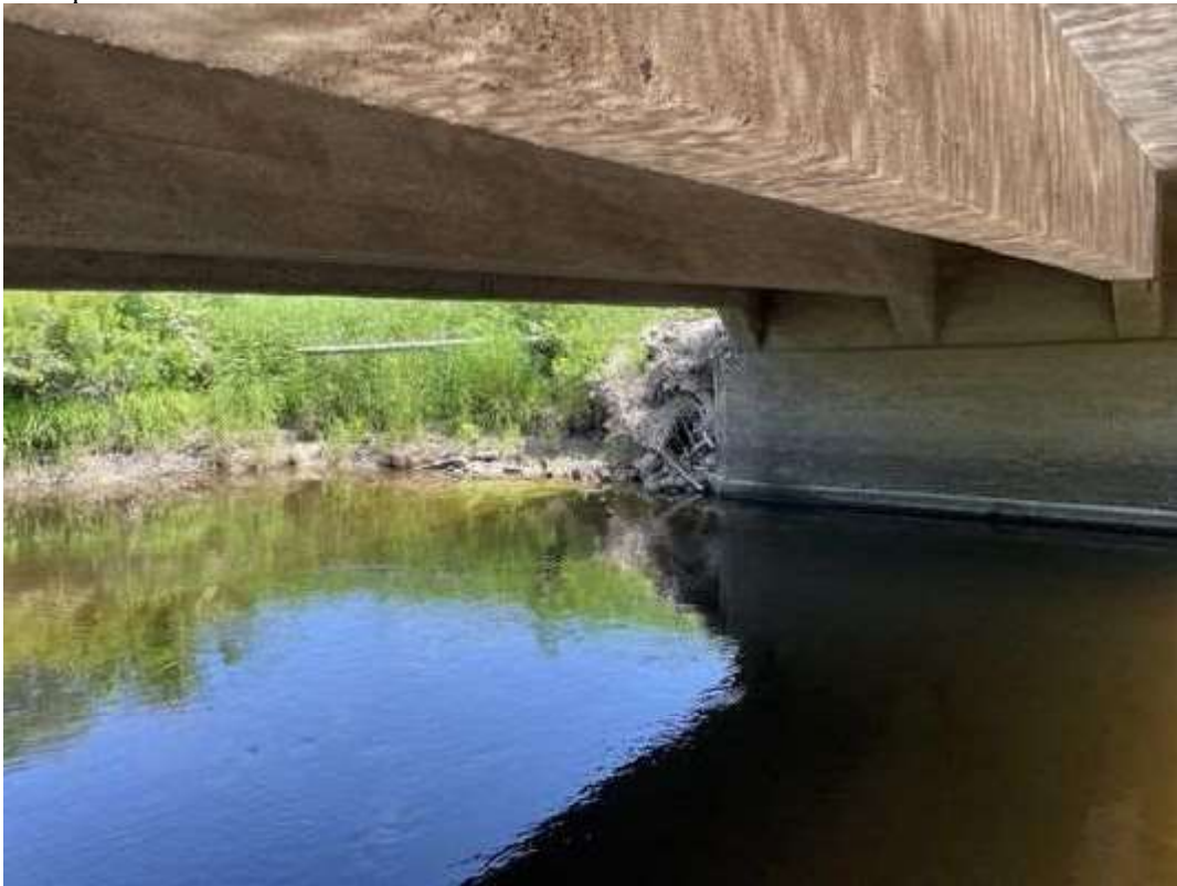
Photo 2: South pier foundation.
