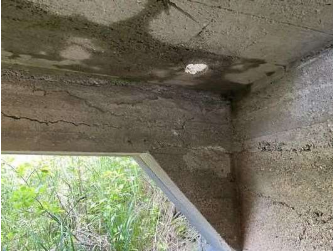
Photo 3: Spall at west side.
