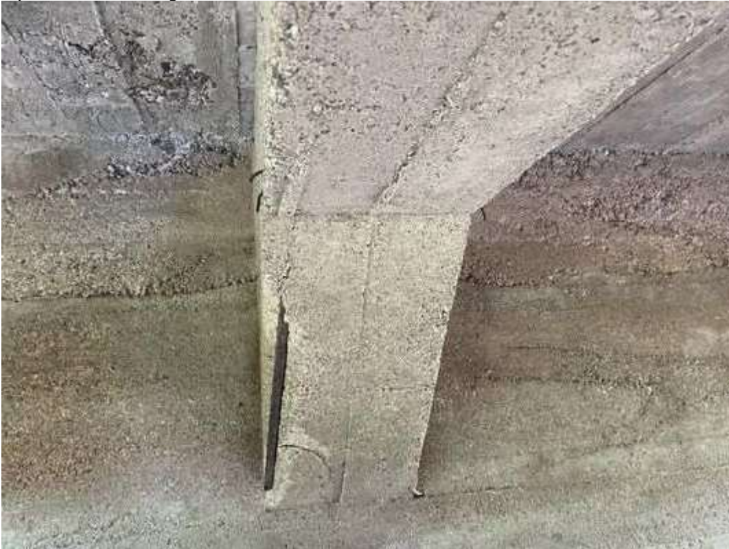
Photo 5: Exposed rebar at south girder haunches.
